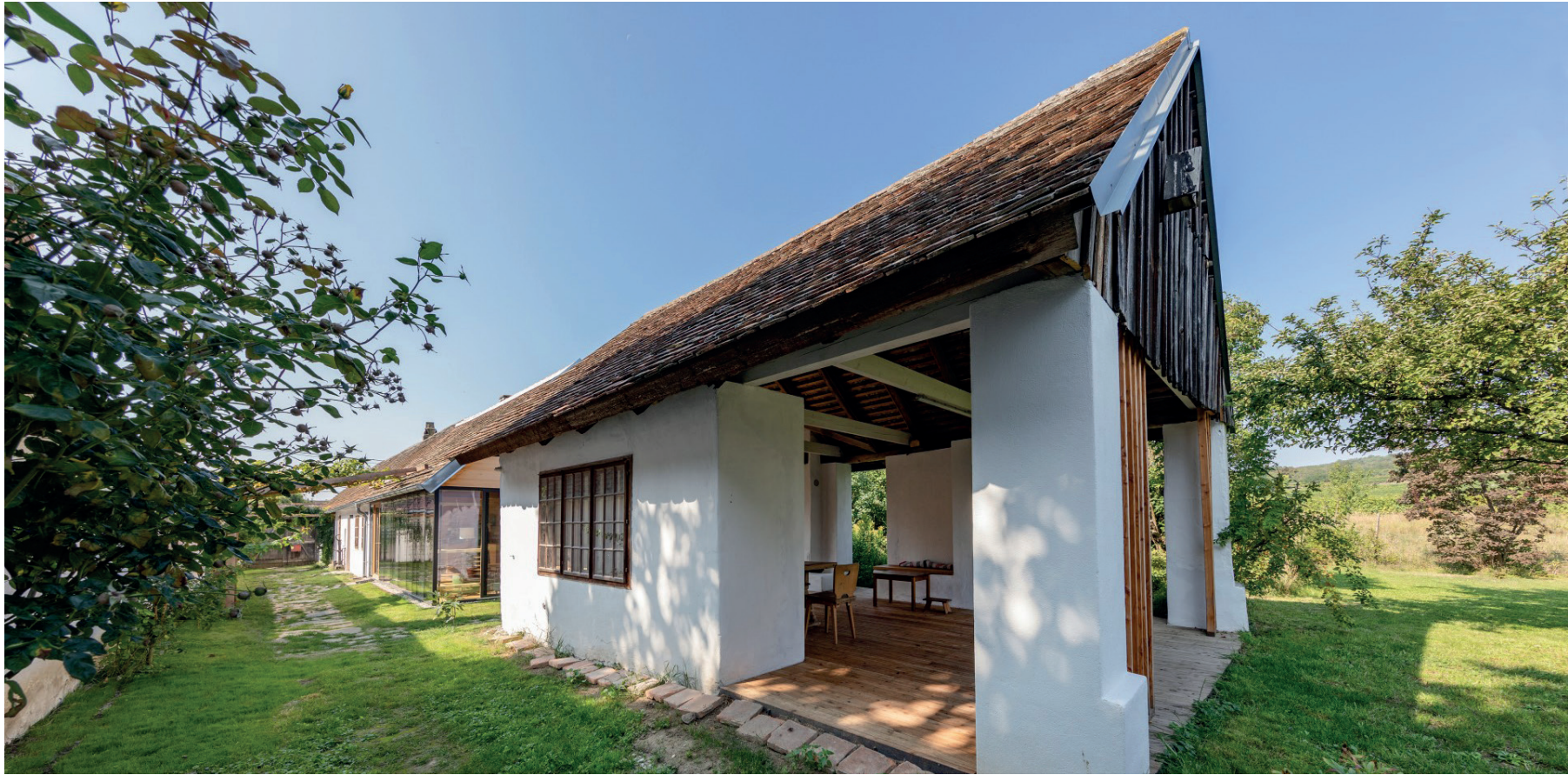
1 noe lehmhaus retzbach
