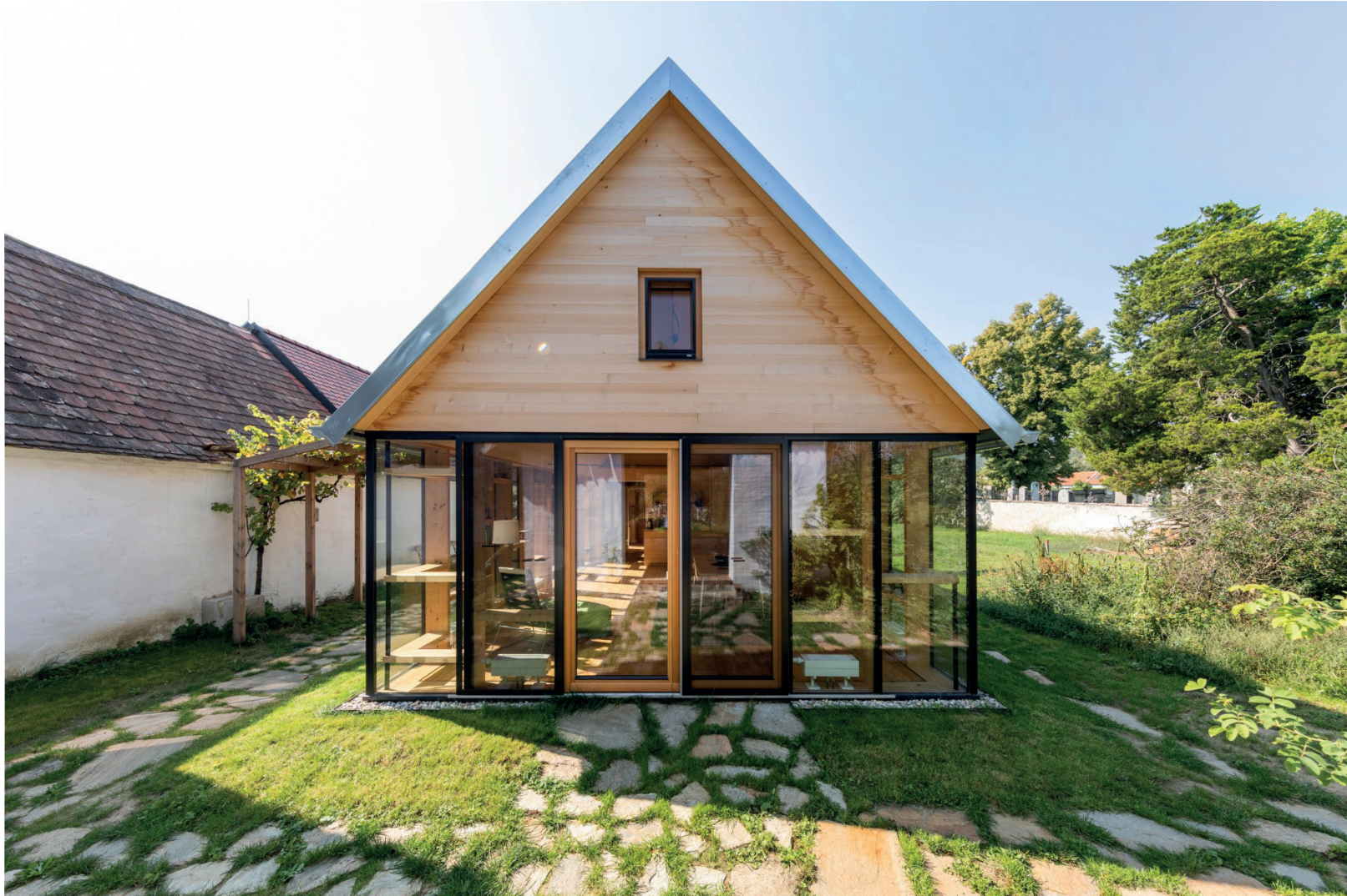
1 noe lehmhaus retzbach
