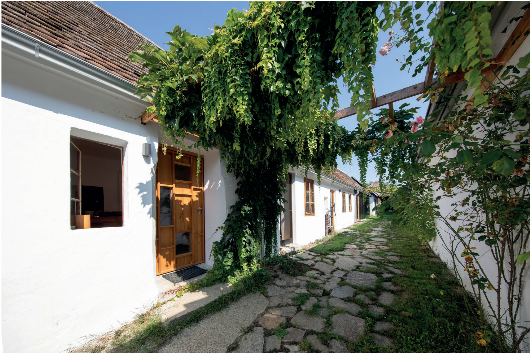
1 noe lehmhaus retzbach
